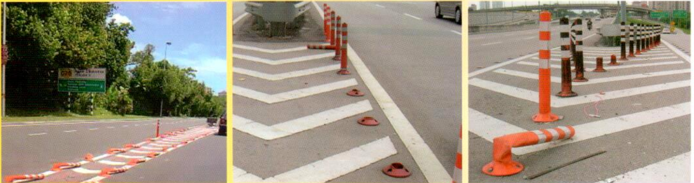
Other reboundable delineators are not able to withstand multiple hits.
